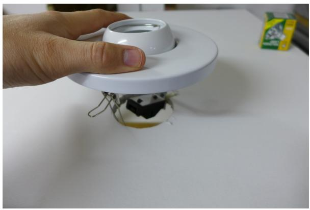
firmly push the fitting into the ceiling, the smaller clips will engage and hold the fitting in place
