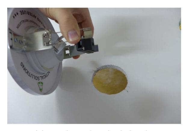
Pinch the spring clips up and towards each other and insert the ends into the hole
